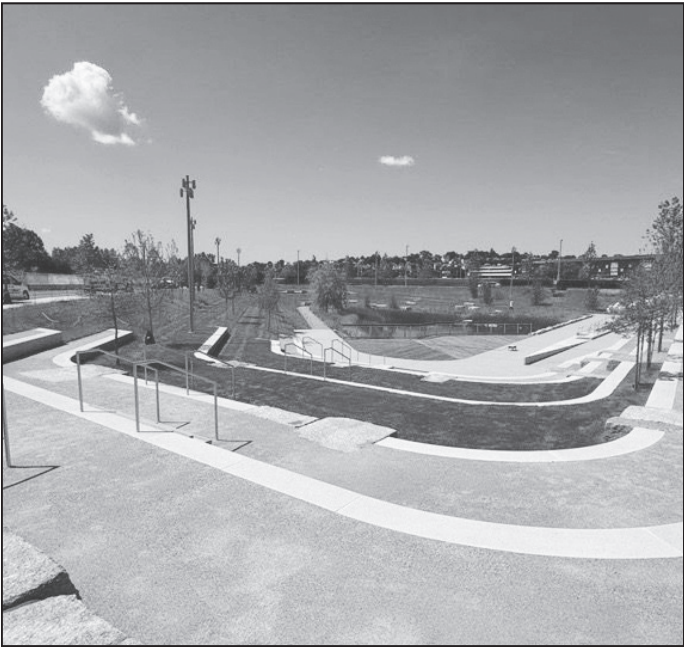
The newly constructed Amphitheater space at Suffolk Downs.
