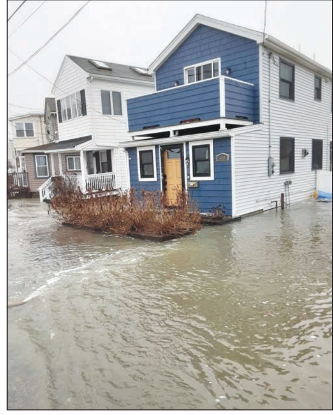
COURTESY OF MASSACHUSETTS RAPID RESPONSE COASTAL STORM DAMAGE ASSESSMENT TEAM
